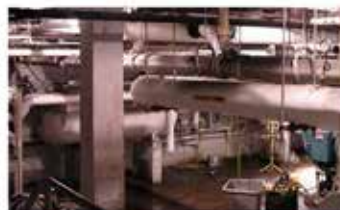
Drenaggio acqua dai locali seminterrati Draining water from the basement
